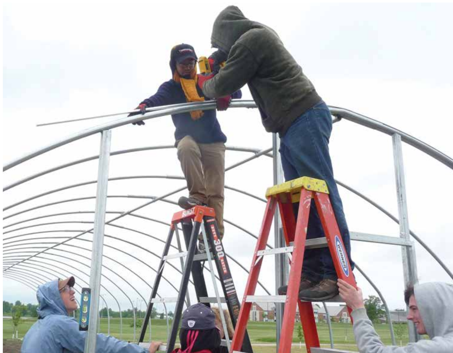
University students construct a hoop house based on a Noble Foundation design.
